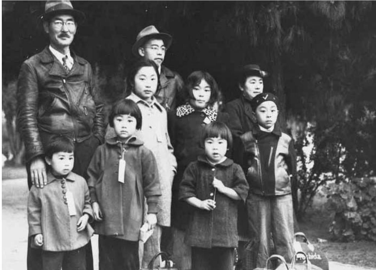
Photo courtesy of the National Archives and Records Administration
